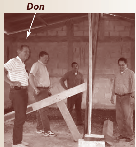
New church building construction by GOLI in Sitio, Guatemala.
